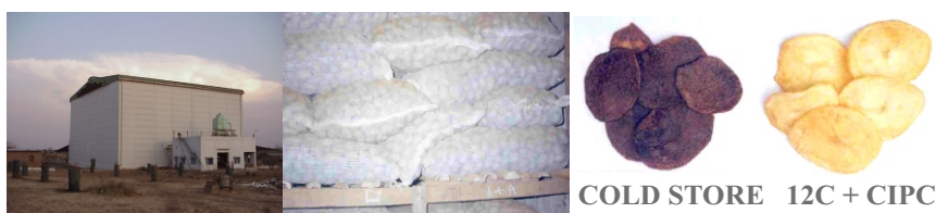
Figure 16: A commercial cold store using 10-12°C storage technology, potatoes stored in leno bags and comparison of chip colour from two refrigerated storages
