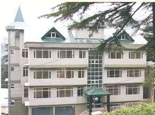
Front view of new building inaugurated by the DG, ICAR
